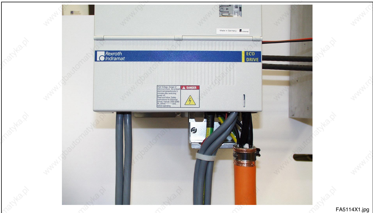
Fig. 16-32: View with contact protection
