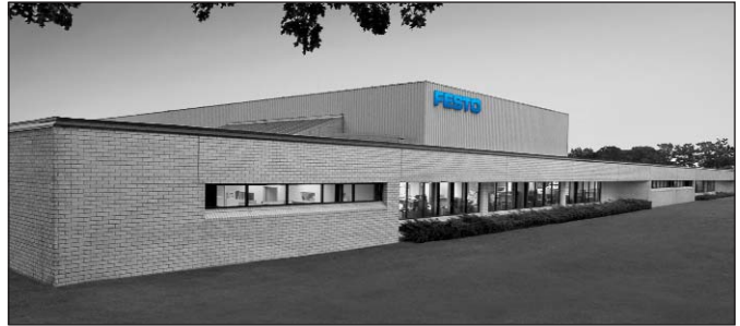
East: 395 Moreland Road, Hauppauge, NY 11788
