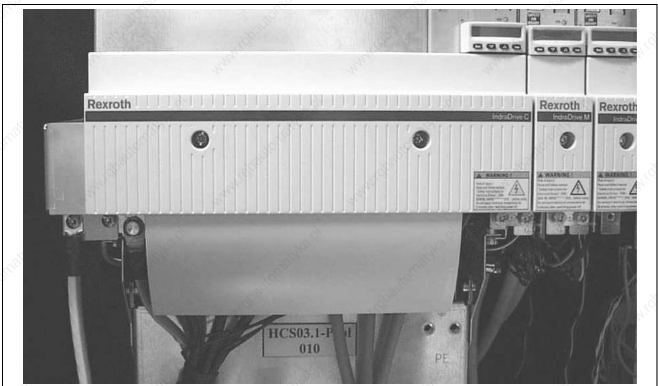
Fig. 14-61: HAS04.1-002 at drive system HCS03 with HMx01 with touch guard mounted
