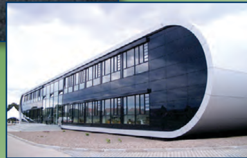
PULS Green Award Winning Plant in Czech Republic
