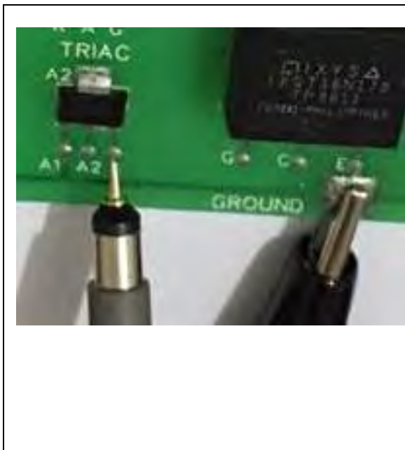
Figure 166: Channel1 Probe Used for Gate - Anode1 Measurement
