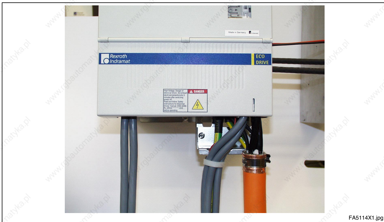
Fig. 16-32: View with contact protection
