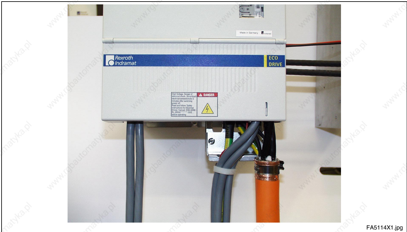
Fig. 16-32: View with contact protection
