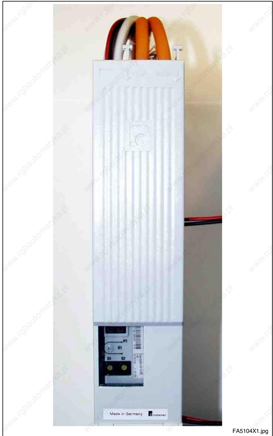
Fig. 16-21: View with contact protection
