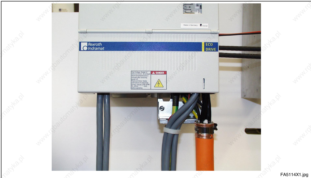
Fig. 16-32: View with contact protection
