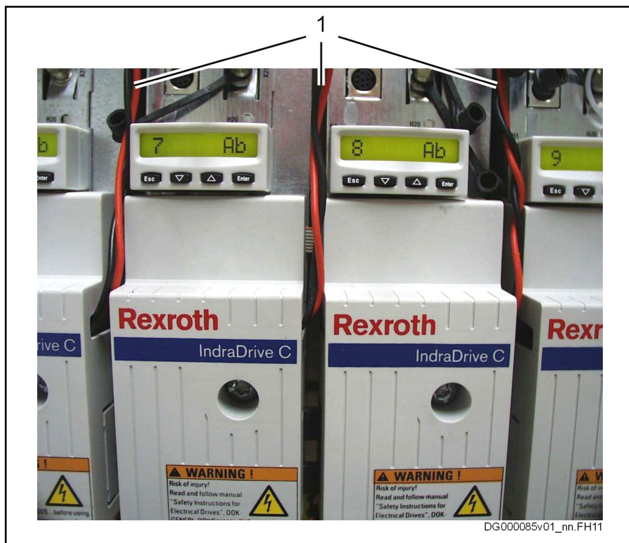
1 Lines to control voltage supply Fig.8-9: Control Voltage Supply at X13
